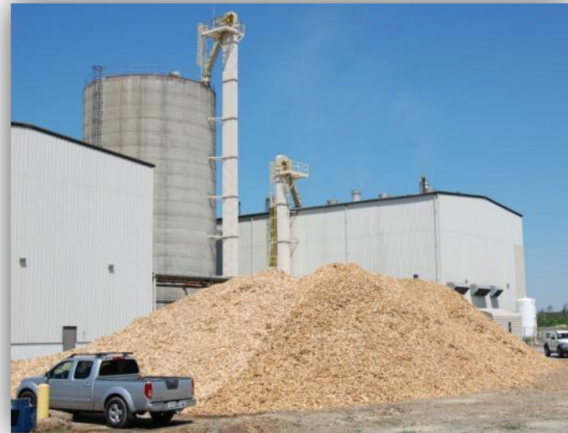
Figure 2.0-5: Wood-based Power Plant
